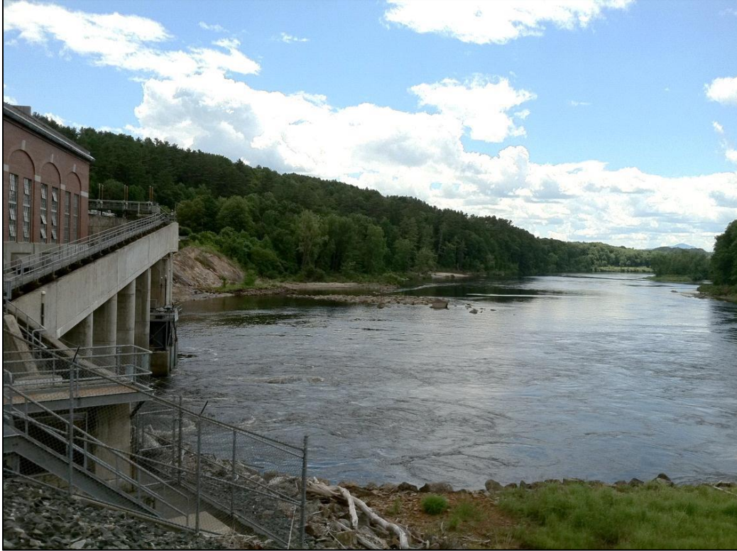
Figure 3.11-1. View downstream of Wilder dam.
