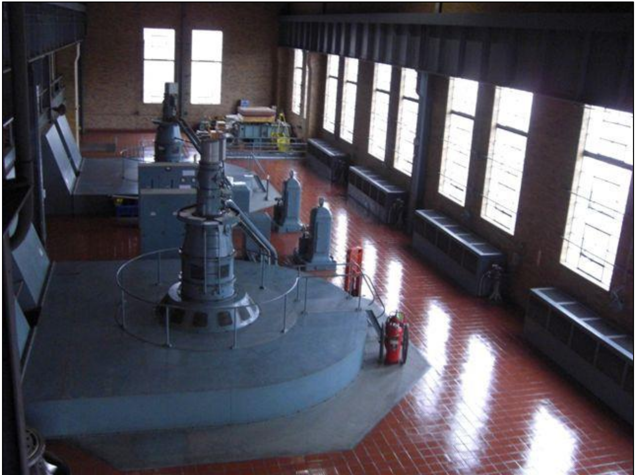
Figure 2.3-3. Generator Units No. 1 and 2.
